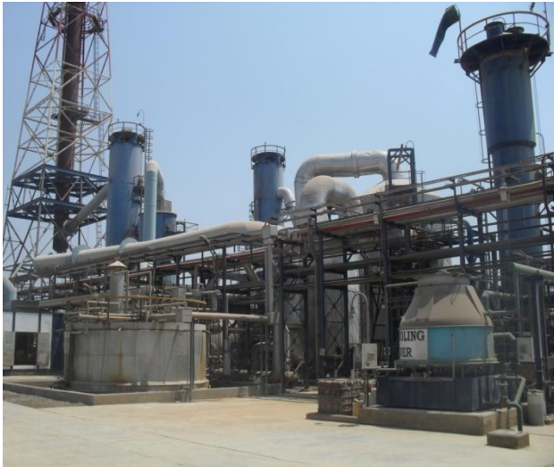
Figure 15 : View of the sulfuric acid plant
