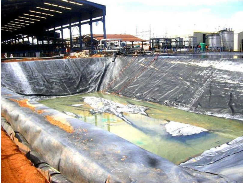
Figure 11 : Geomembrane depleted electrolyte pool
